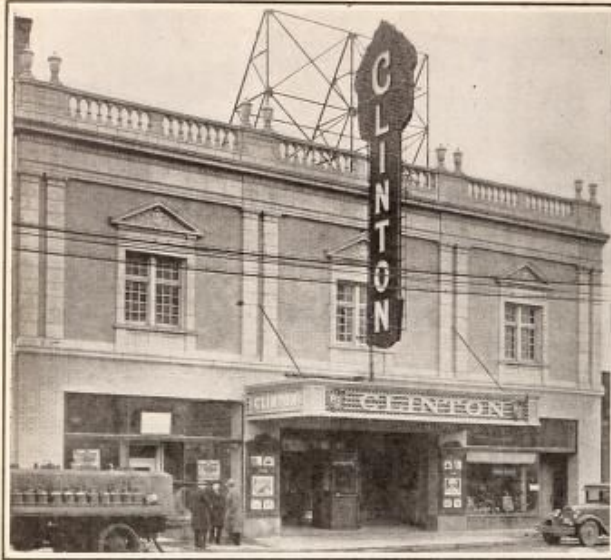
The Clinton Theatre, Columbus, O., equipped with air conditioning system. The Clinton is a 1500-seat house and is one of the many theatres with less than 2000 capacity having this equipment.
